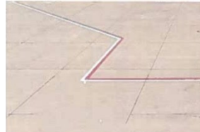
Apron Safety Lines
