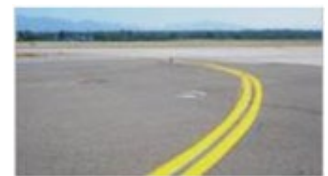
Taxiway Edge Markings
