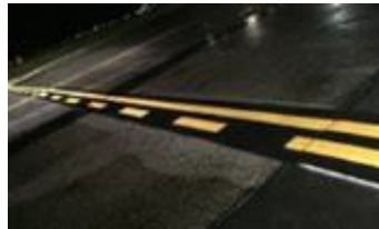
Manoeuvring Area Delimitation Line
